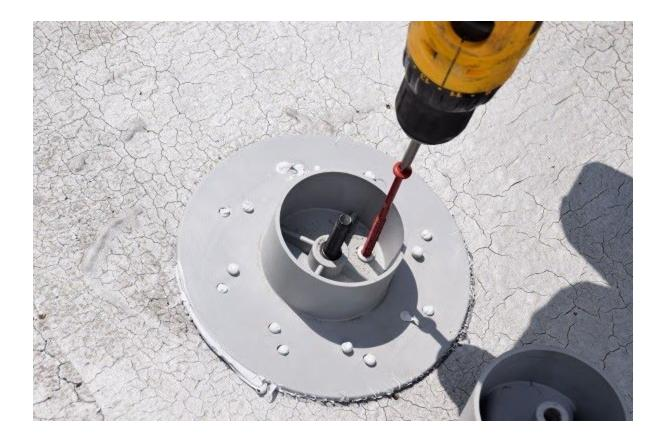
STEP 6 (OPTIONAL) INSTALLING EXTENSIONS If the installation is to be elevated, slide the appropriate extensions into the base.
