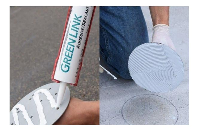
STEP 4 (OPTIONAL) PLACEMENT OF THE BASE Position the base in the marked area and press gently. GREEN LINK Adhesive/Sealant should squeeze out from the "rivet holes."
